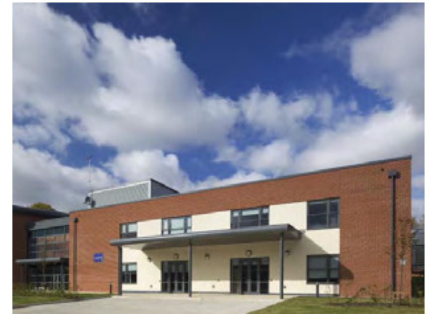
Above: Training facilities at Tidworth
